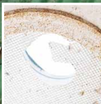
One of John's plastic dome skylights from the inside: hail stones crashed right through. ▲
