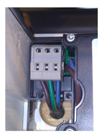
The Wago plug is located on the left hand side of the electric operator.
